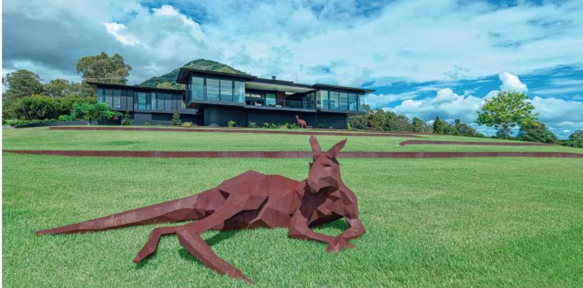
The 2019 Master Builders Queensland House of the Year winner was the Cooroy Mountain Residence by Braeden Constructions.
